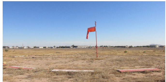
Lighted Wind Cone and Segmented Circle
