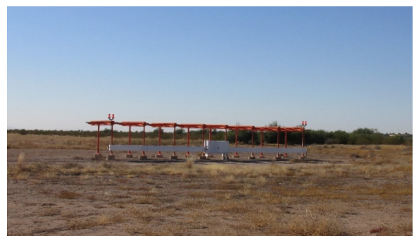
Localizer Antenna Array
