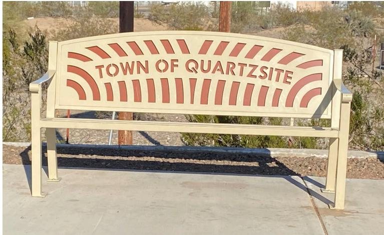
Benches shall be surface mounted per the manufacturer recommendations on a 4-inch thick concrete pad. The color of the concrete pad shall match the color of the adjacent sidewalk. Concrete pad shall extend 3" beyond the bench legs as detailed on the plans.
